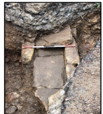
A culvert under Durham's Market Place: or a tunnel, if you're a ferret.
