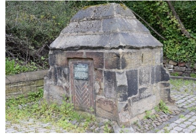
The old Fram Well Head, re-erected near the railway in 1959.
