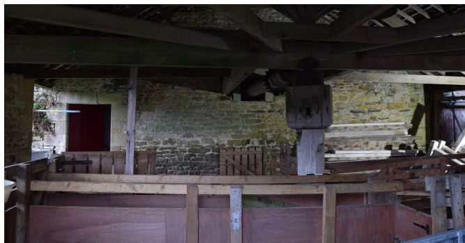
A rare example of a gin gang where the drive shafts survive. The horizontal shaft enters the barn through a square hole at the middle of the picture.
