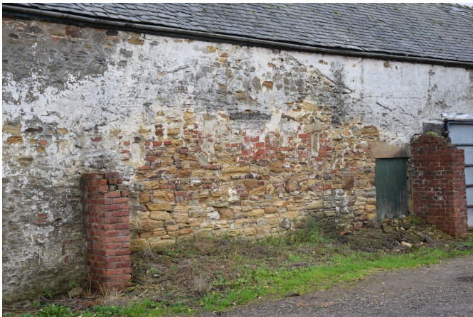
A barn on the edge of Durham City. The line of the low-pitched roof of a vanished wheelhouse can be seen under the whitewash.
