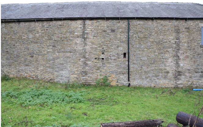
In this barn at Kepier, just outside Durham, traces of the gin gang are harder to spot, but the door and the central holes give its former presence away.
