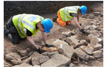
PCA Durham team cleaning the foundations for the north wall of the turret. © Pre-Construct Archaeology
