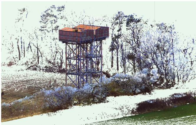
Figure 2. Point cloud capture of redundant water tower, Tranwell, near Morpeth.
