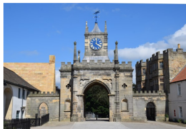
Refurbished Robinson Arch.
